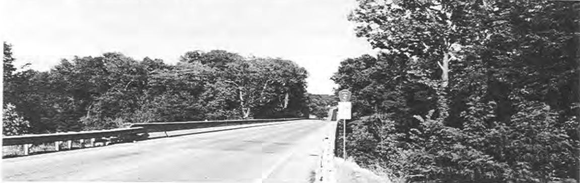
New Salem Bridge
