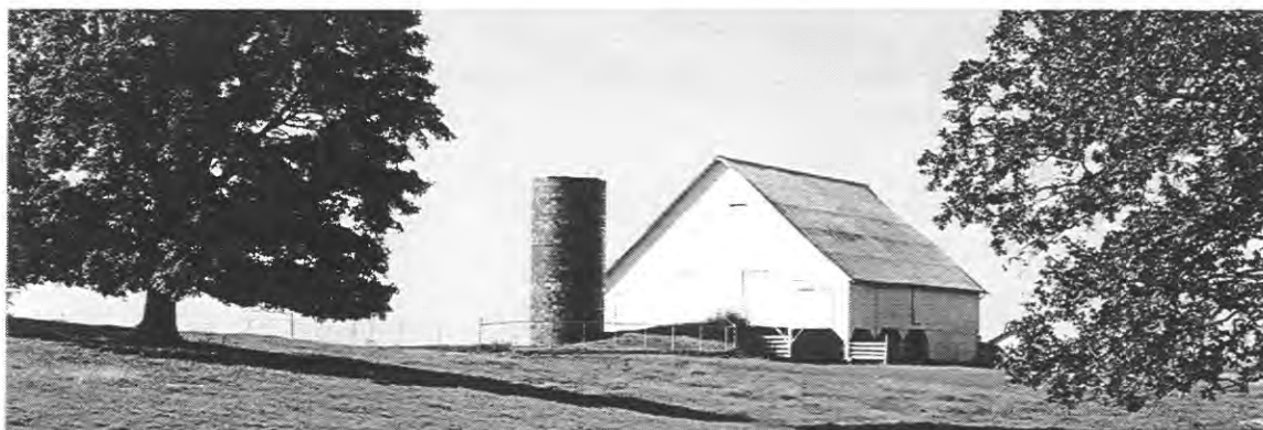
Barn and Silo on Rock Creek Road
