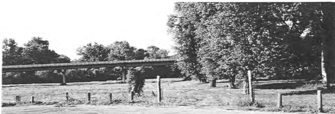
Old River Road at Petersburg's Bridge Park
